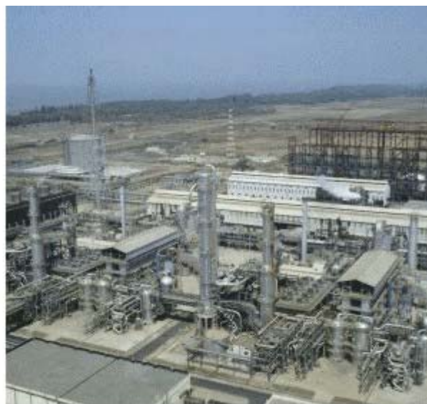
Ammoniak-Anlage in Bombay, Indien (C) Poul Møller, Haldor Topsøe A/S, Denmark
